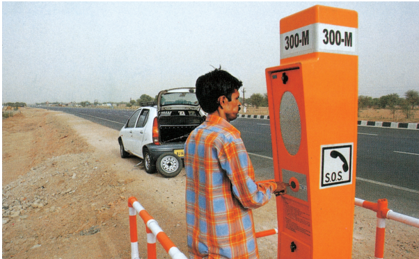
Fig. 7.10 : Emergency call box on NH-8
